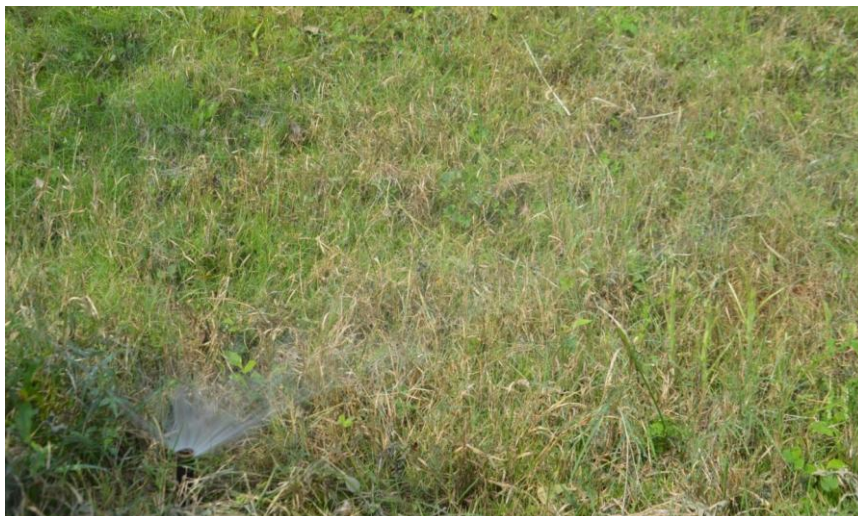
Sprinkler Irrigation System
